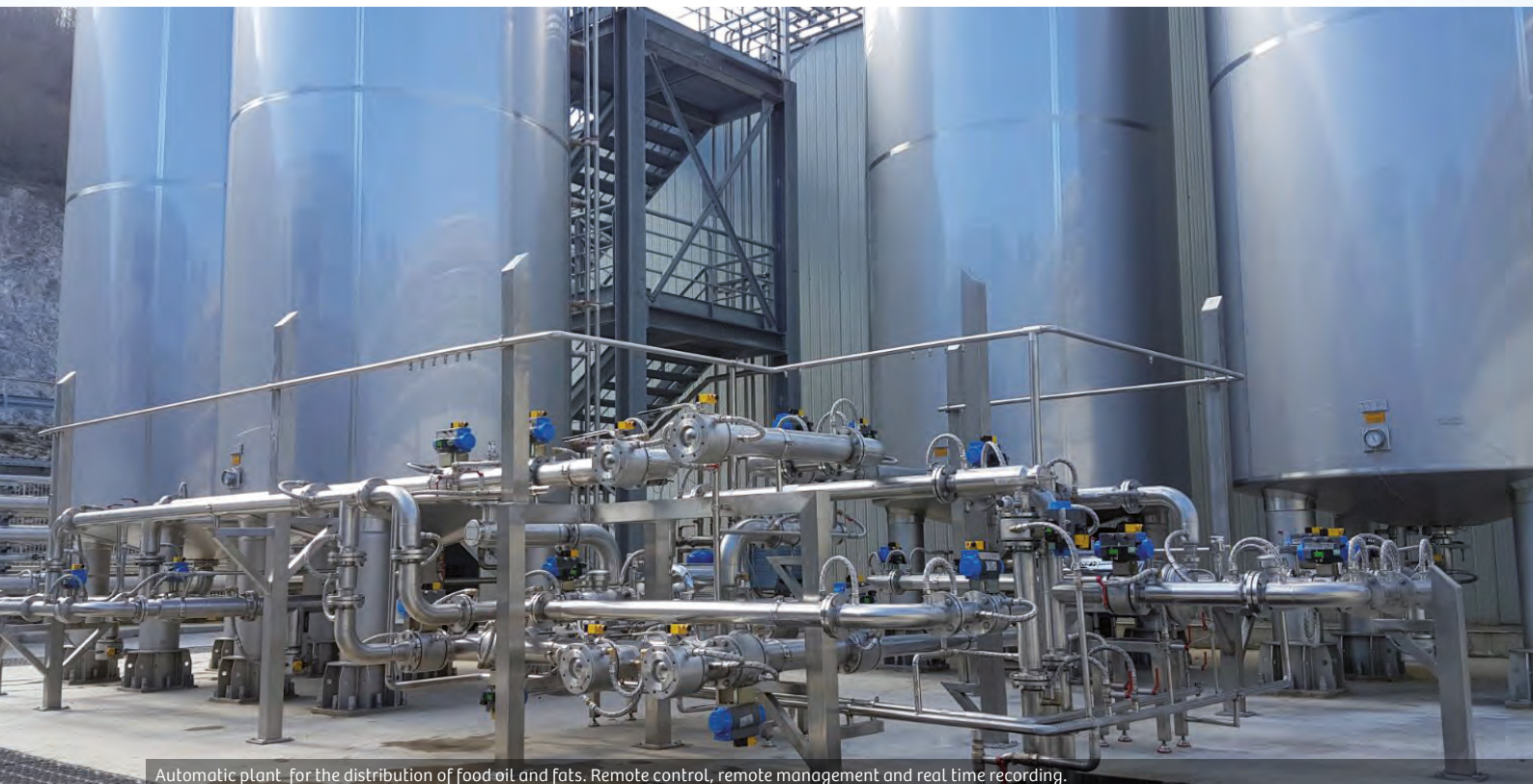
Automatic plant for the distribution of food oil and fats. Remote control, remote management and real time recording.
